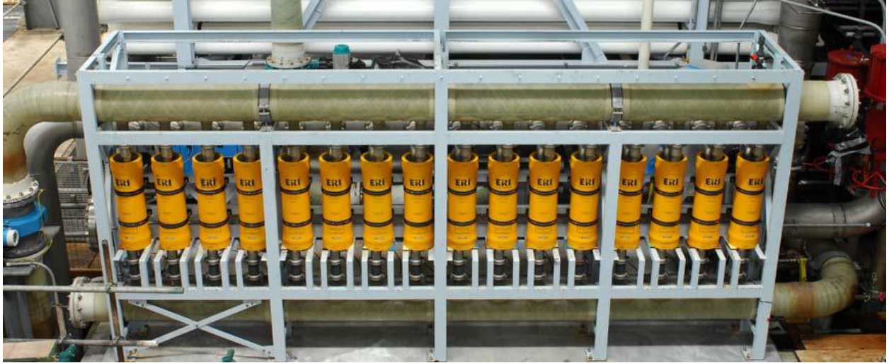
Fig 2.13: PX Device Array Serving SWRO Train 6A Perth, Australia (Sanz and Stover, 2007).
